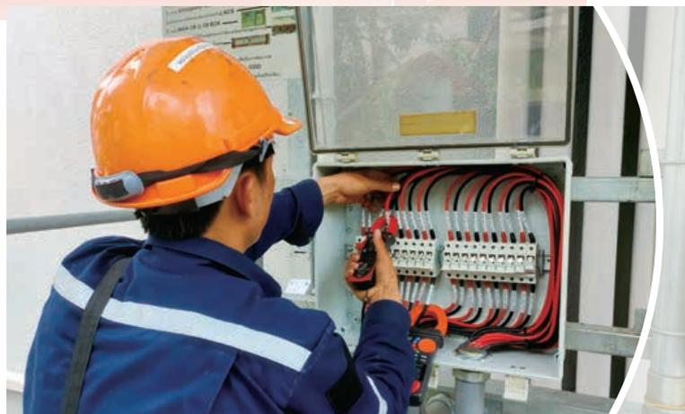
An RPCL worker performs preventive maintenance fuse checks for a solar rooftop project at an administration building.
