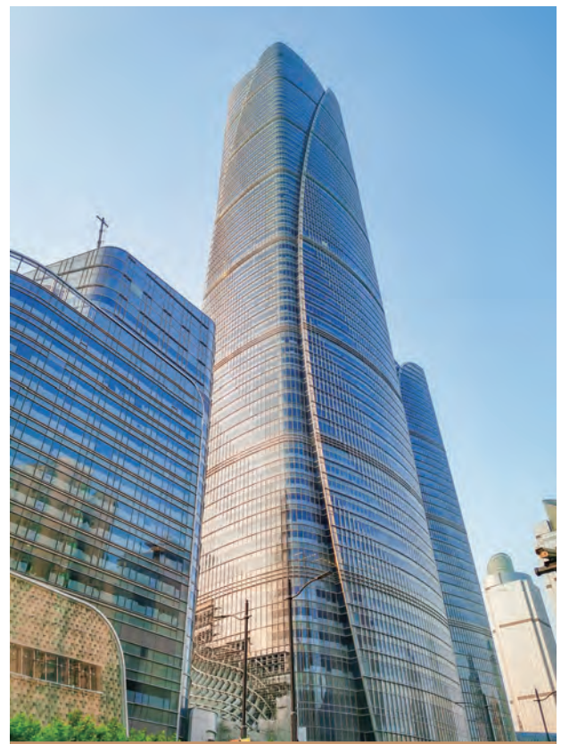
○ Tower B of Three ITC, Shanghai
